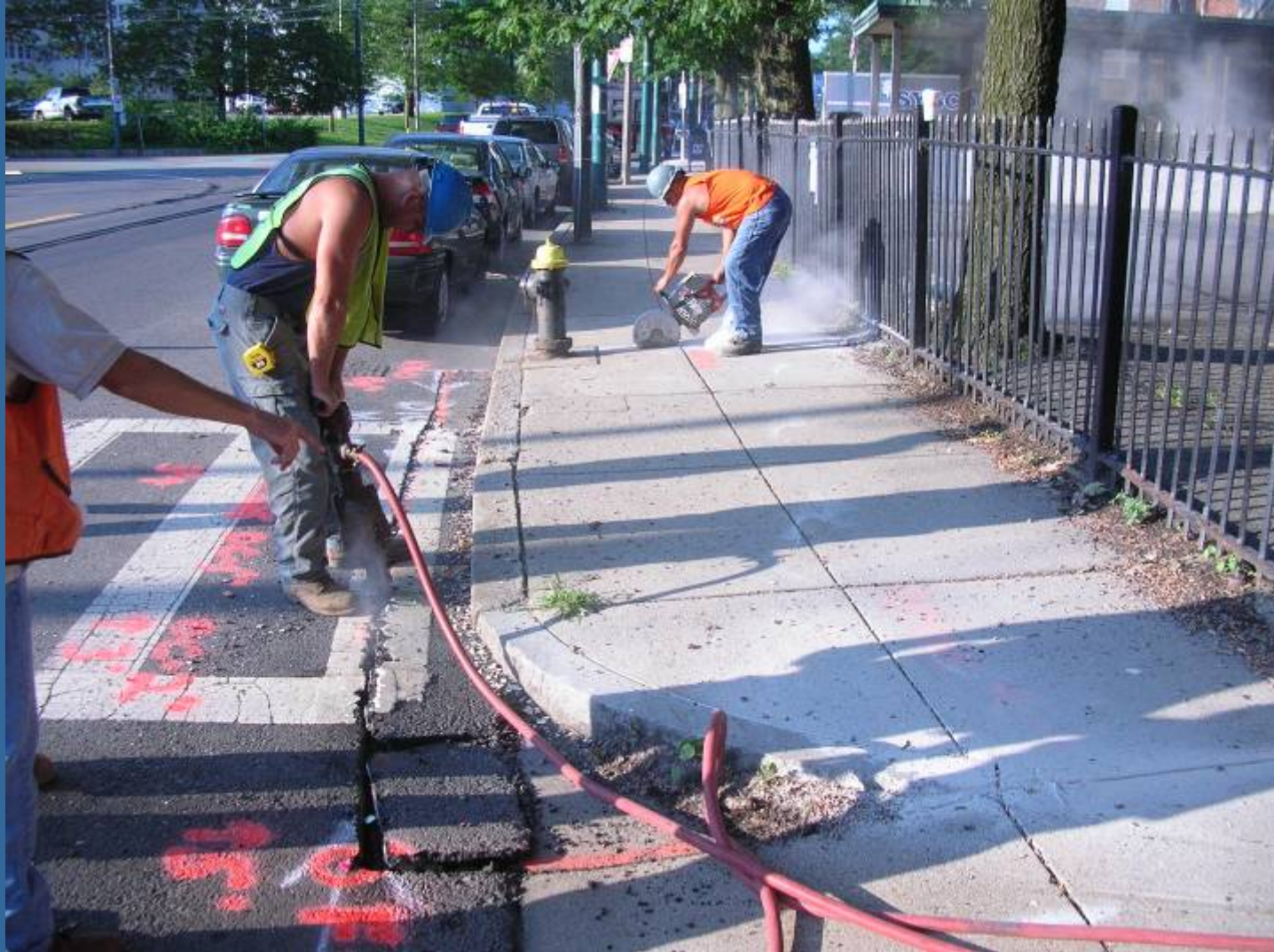
Sawcut Pavement and Sidewalk
