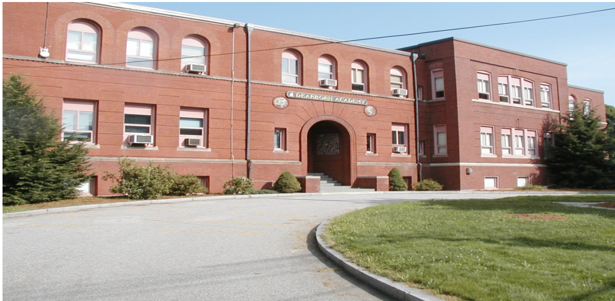
Figure 1 – Exterior View of the Crosby School in Arlington, MA
