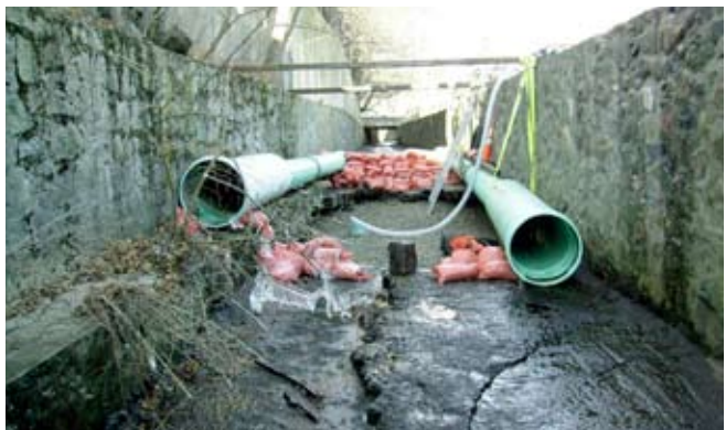
Emergency repair site of Mill Brook Culvert by Ryder Street.
