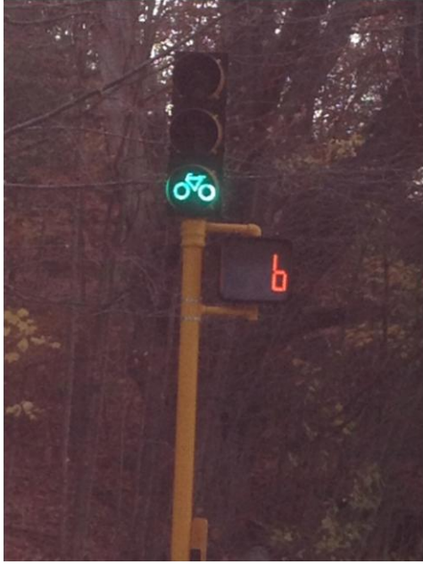
Figure 1 Bicycle/Pedestrian Signal (Minuteman Bikeway/Bedford Street Lexington, MA)
