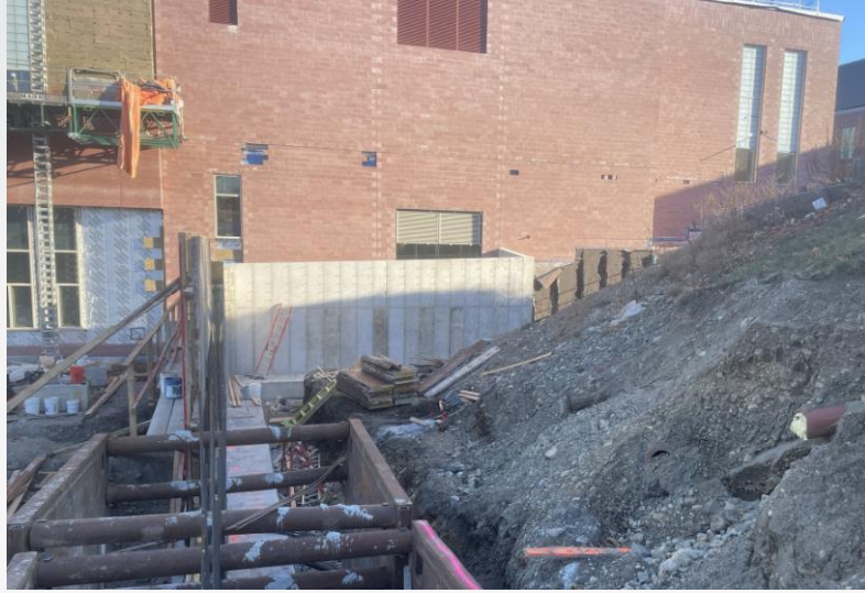
Building A – West Retaining Wall Work
