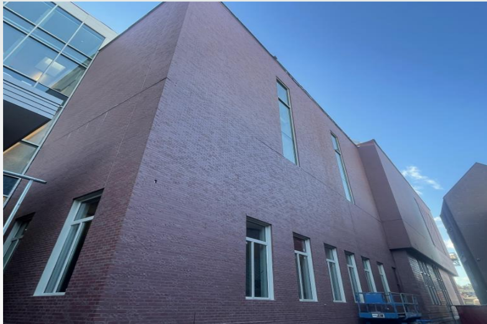
Exterior Building A - North
