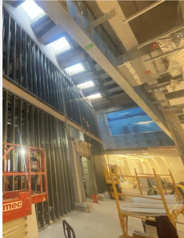
PH 2 + 3 Tie In Point
