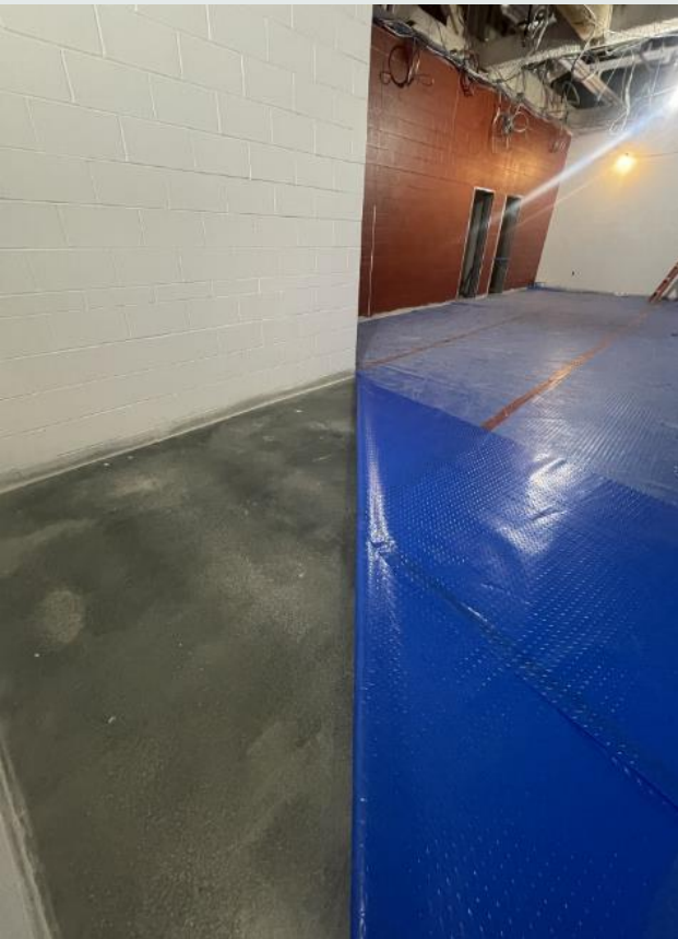
Locker Room Polished Concrete + Painting
