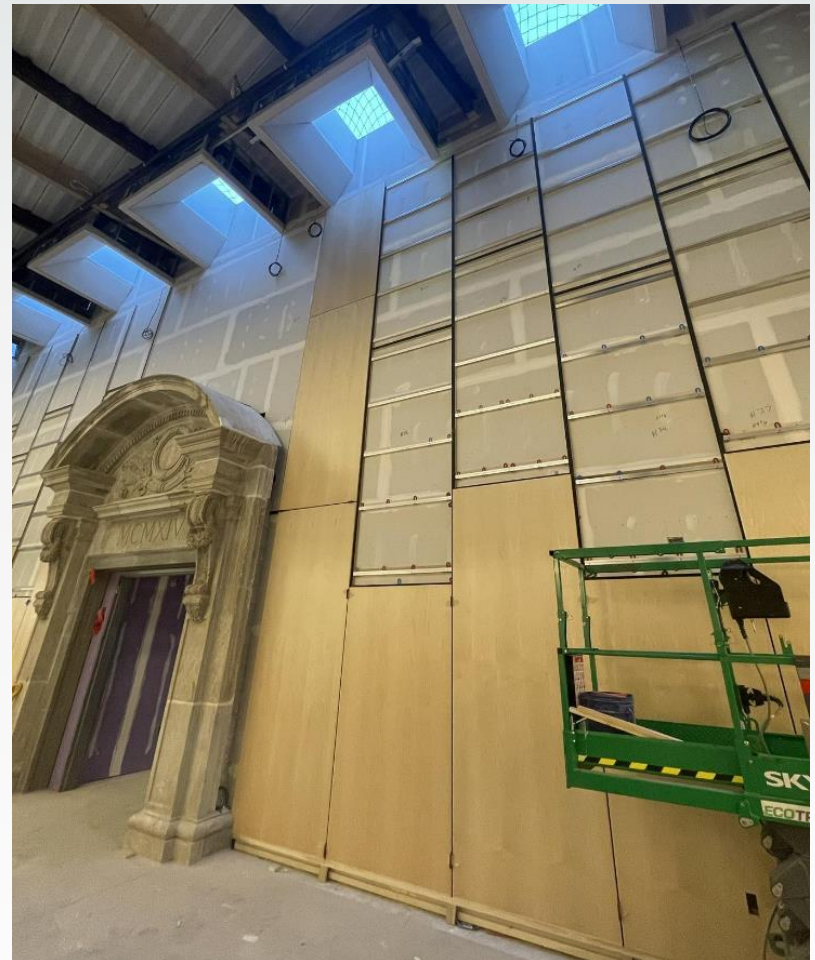
Salvaged Masonry + Wood Paneling
