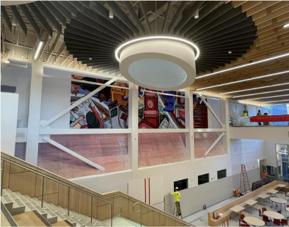
PH 2 + 3 Tie In Point (Terrazzo Install)
