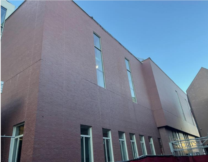
Exterior Building A - North
