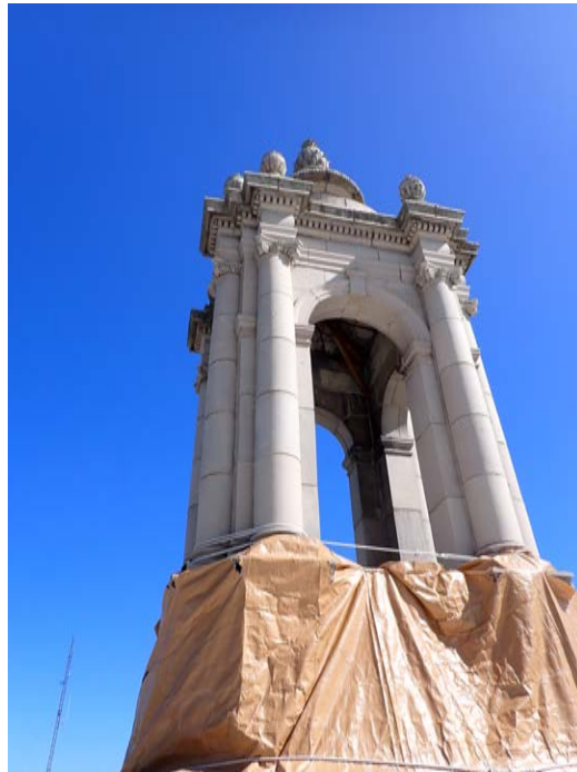
Figure 1. Cupola above podium.
