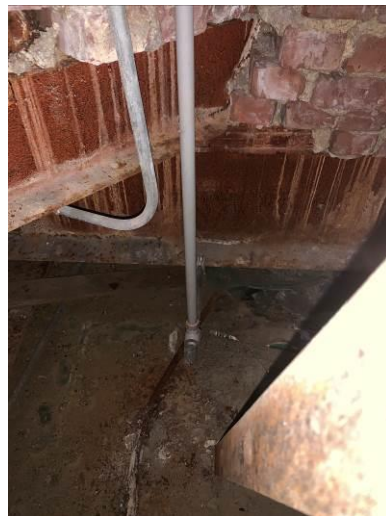
Conduit and Wiring at Lower Tower
