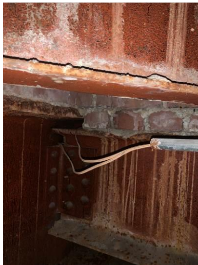
Conduit and Wiring at Lower Tower
